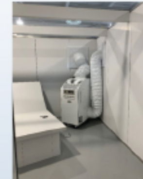
Figure 7: Room After Installation for Positive Pressure
